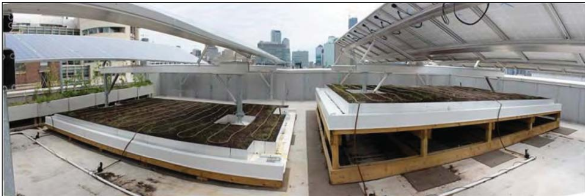
Figure 4: Completed Phase II GRITlab.
