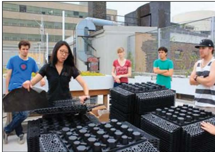
Figure 5: Student training by industry partner Bioroof Systems on green roof module assembly
